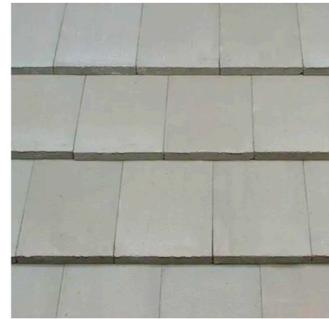
CEMENT TILE ROOF
