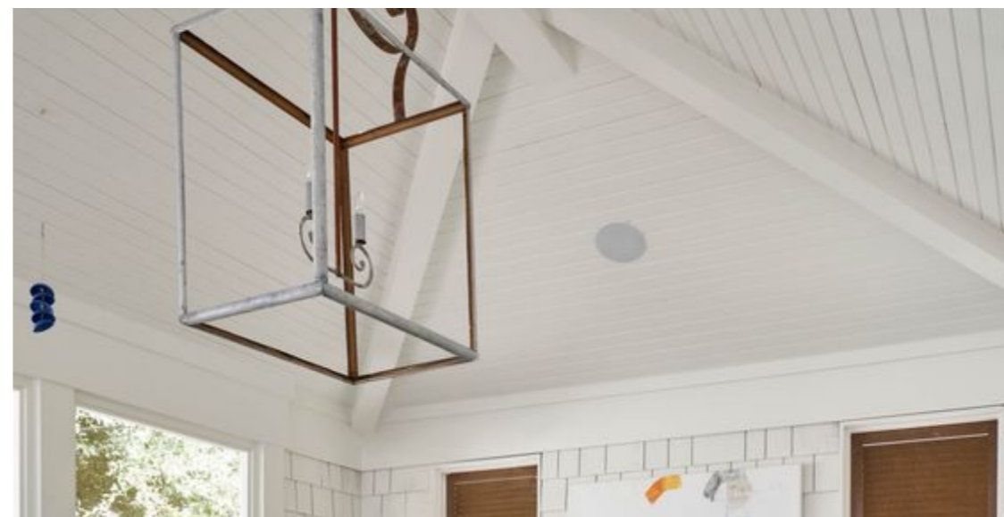
FAMILY ROOM VAULTED CEILING WITH DIME JOINT
