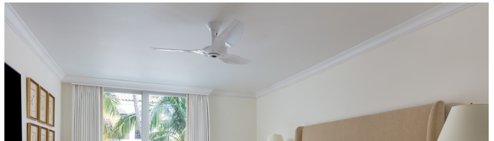
DRYWALL CEILING WITH CROWN
