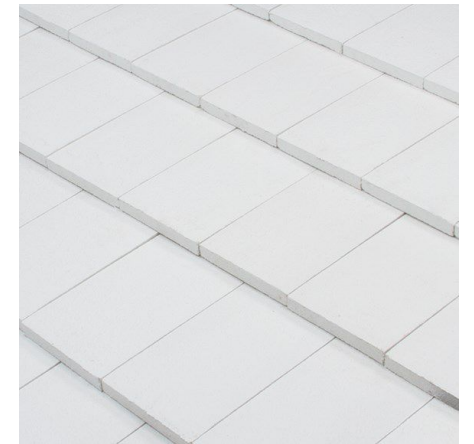
WHITE TILE ROOF
