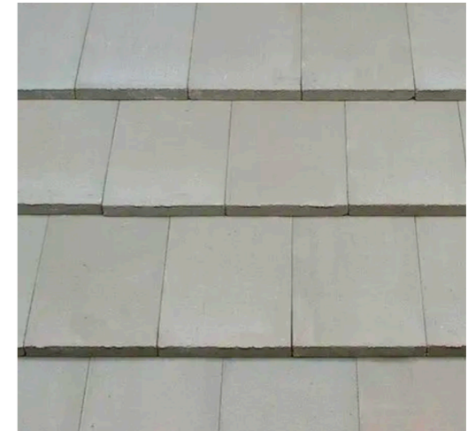
CEMENT TILE ROOF
