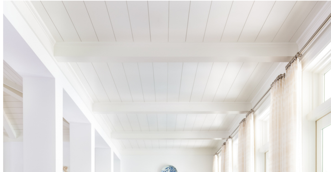
WHITE T&G CEILING WITH BEAMS
