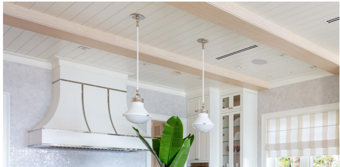
DIME JOINT CEILING WITH OAK BEAMS
