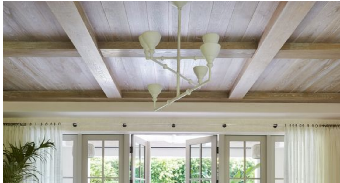
LIVING ROOM COFFERED CEILING WITH DIME JOINT
