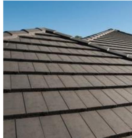
GRAY CEMENT TILE ROOF
